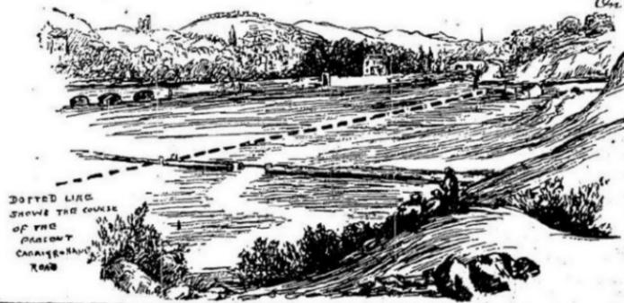
to the West by the old Ballincollig road became congested and a new-line from Victoria Cross to Carrigrohane commenced about 1840. Giving to the swampy nature of the land, foundations for a road-bed and substantial disches were constructed to protect from flooding on the north by the Lee, and on the South sy the Maglin river which flows through marsky ground for a considerable distance.
